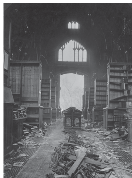
Bomb damage to the Victorian library, 1940
